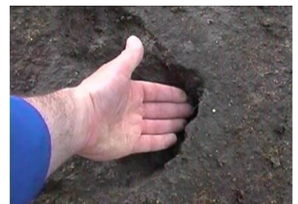
Hole in the floor resulting in lame pigs
